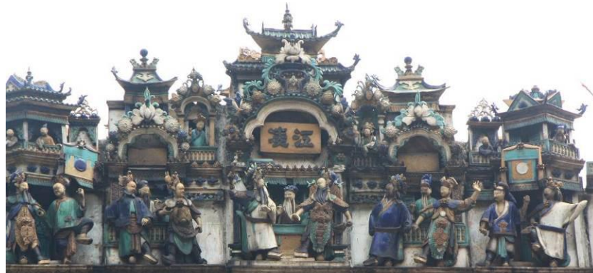
Fig. 11 Ceramic ridges in Chen Clan Academy (photographed by Lv Tangjun)
