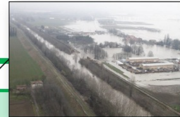
Typical embankment enforcement
